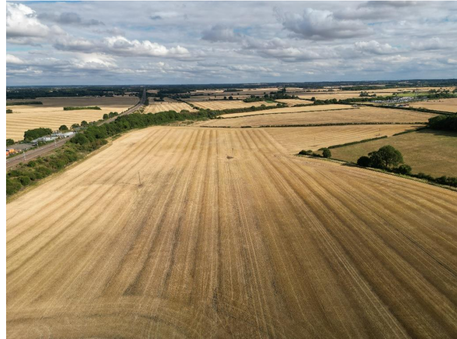
Photo below: The fields west of the ECML, Field 26 foreground, followed by Field 18 and then 19 the right of the shot shows the corner of Freeward wood with the current Ryhall substation and the ECML Essednine substation on the left.
